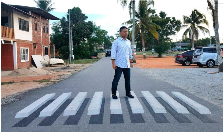
Image 3: The 3D zebra crossing is an urban intervention that emerged in India. It creates the optical illusion of an elevated pedestrian crossing, stimulating cars to slow down as they approach.
